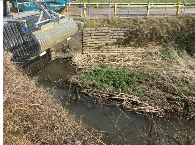
Photo 5: Weir structure upstream of culvert
