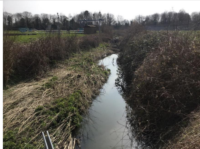
Photo 4: Upstream view from weir, berm formed on right bank narrowing channel
