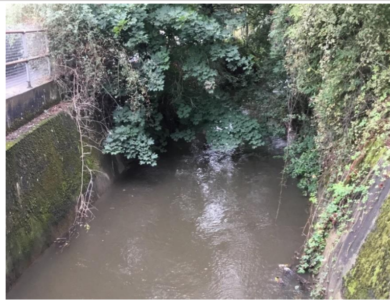
Photo 66: Concrete vertical walls on approach to South Terminal culvert
