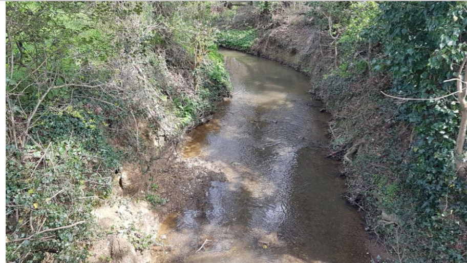
Photo 126: Downstream view from bridge showing steep to vertical bank profile
