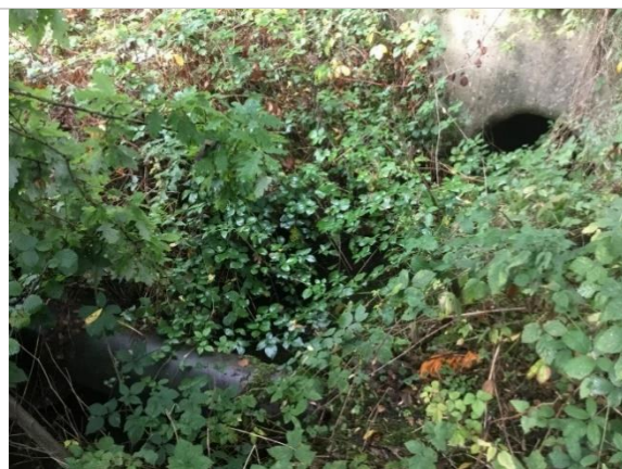
Photo 2: Pipe crossing close to culvert
