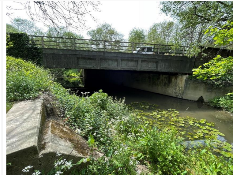
Photo 33: Downstream side of London Road bridge
