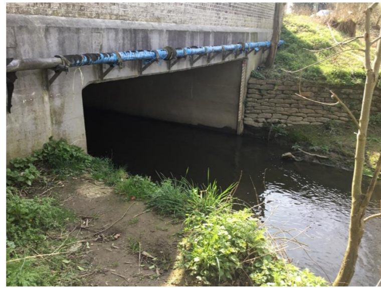
Photo 38: Downstream side of Brighton Road bridge
