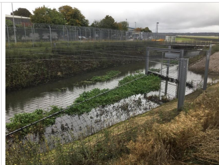
Photo 90: Vegetated mid channel bars adjacent to gated slipway into channel (submerged)
