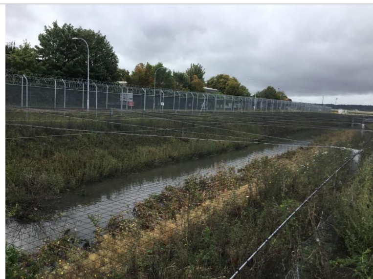
Photo 88: Straightened planform, appears over-deepened. Bird netting covering channel
