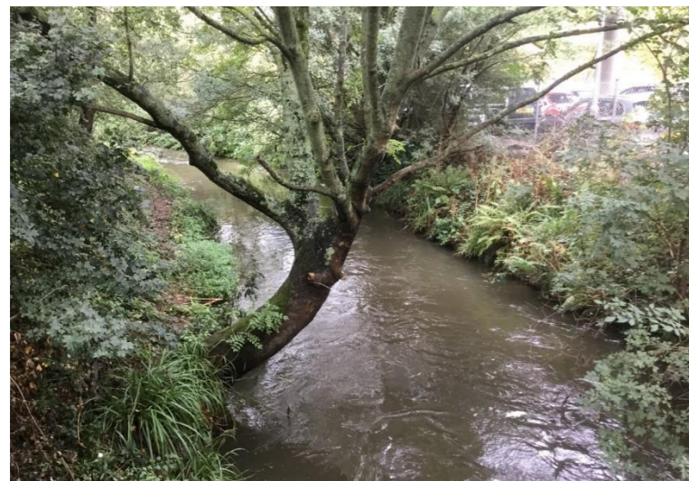
Photo 69: Downstream of South Terminal culvert outlet
