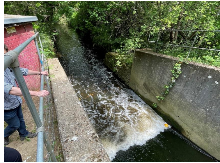
Photo 73: Downstream of Airport Way culvert
