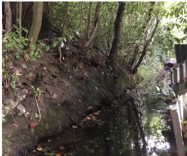
Photo 115: Downstream of culvert along Balcombe Road, heavily shaded, no perceptible flow
