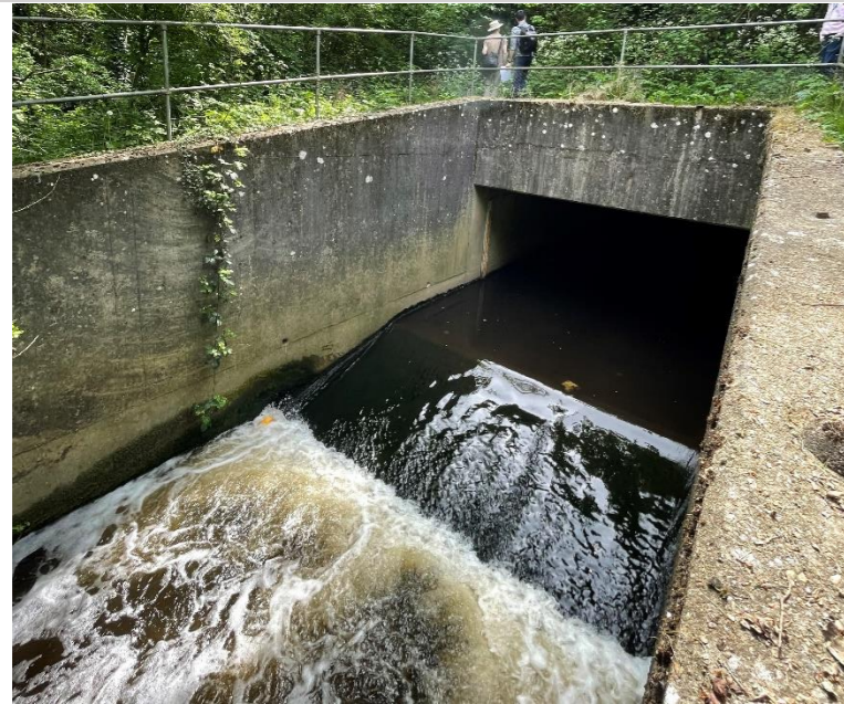
Photo 72: Airport Way culvert outlet and weir structure
