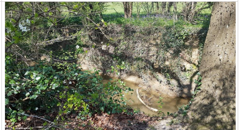
Photo 134: High vertical root-bound banks and turbid water. Flow is perceptible.
