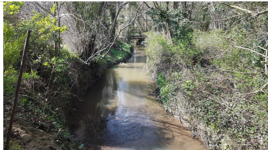
Photo 129: Upstream view toward wooden footbridge from smaller road crossing. Channel is wider and shaded by vegetation. Flow is perceptible.
