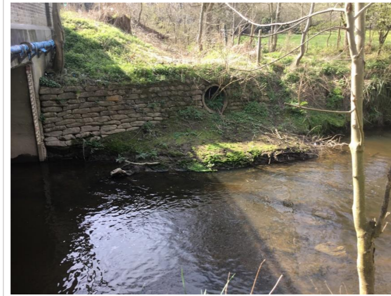
Photo 39: Dry ditch outfall on left bank immediately downstream of Brighton Road bridge
