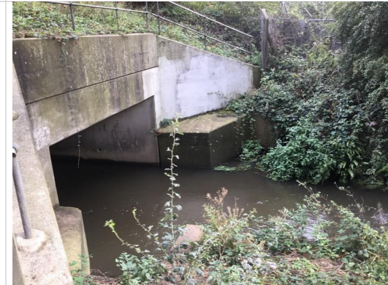
Photo 71: Culvert inlet under Airport Way and London Gatwick Airport shuttle line (outfall on right bank, view obscured by vegetation)
