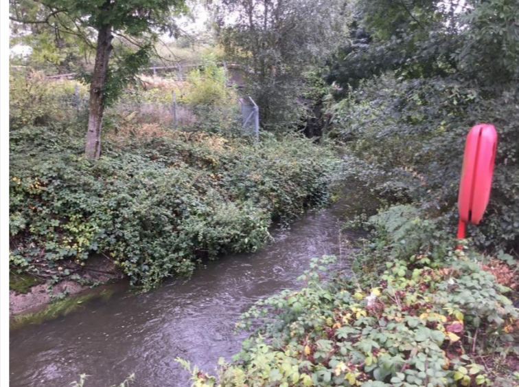
Photo 57: Gatwick Stream passes under the Brighton Main Line railway
