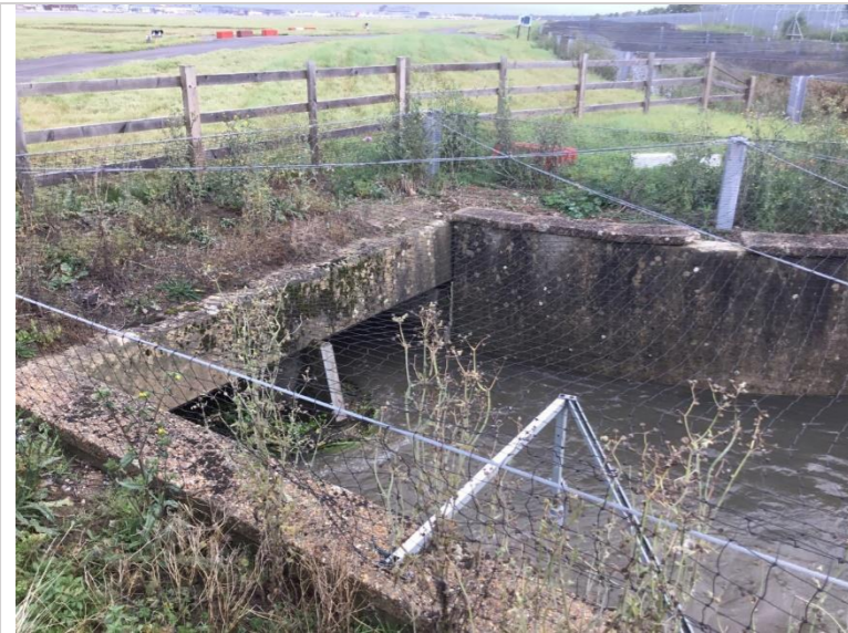
Photo 7: Runway box culvert inlet and divider wall
