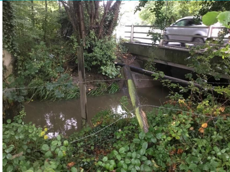
Photo 44: Radford Road bridge at furthest upstream extent
