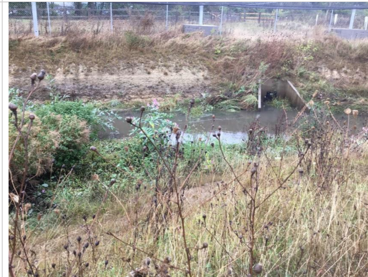
Photo 52: Outfall with concrete headwall on right bank
