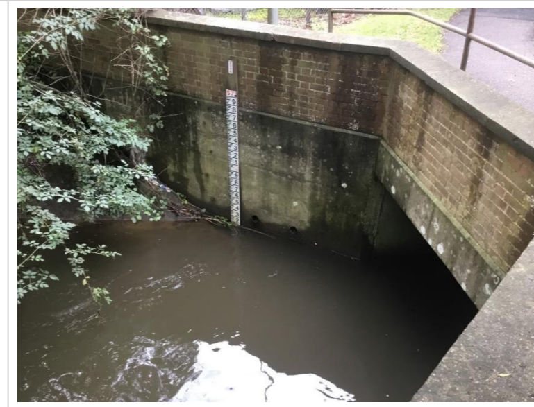
Photo 68: South Terminal culvert outlet
