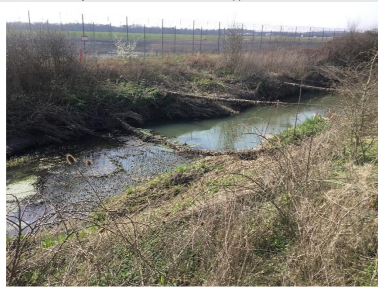
Photo 11: Straightened section of River Mole and old netting impeding flow
