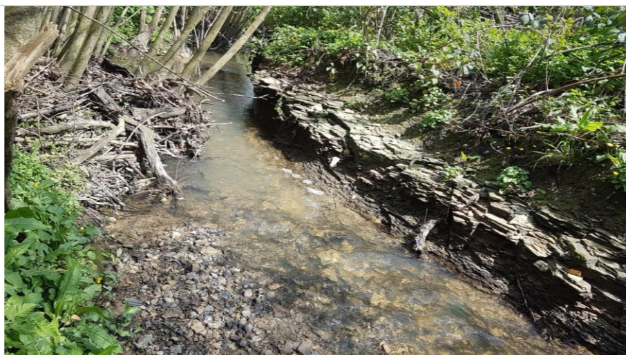
Photo 142: Large gravel bar and bed substrate. Natural wood deflector and narrowing of channel. Mudstone bedding on right bank.
