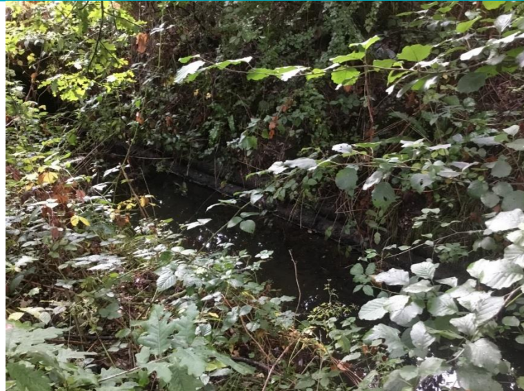
Photo 112: Concrete lined channel upstream of culvert, heavily shaded
