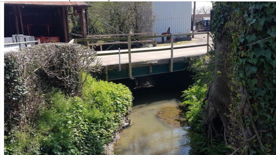
Photo 130: Road bridge set into vertical bank face
