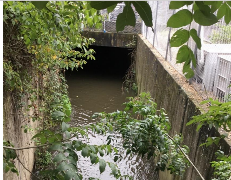
Photo 67: South Terminal culvert inlet
