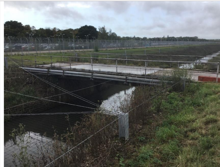
Photo 107: Access bridge and concrete abutments
