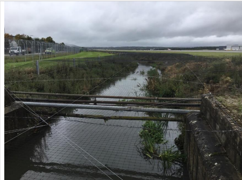
Photo 94: Multiple pipe crossings downstream of concrete access bridge
