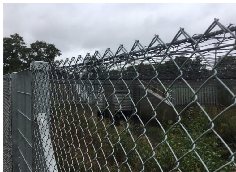
Photo 56: Channel feeds through wastewater treatment plant infrastructure
