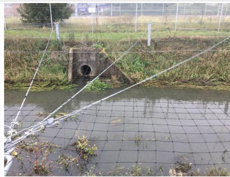
Photo 101: Concrete outfall on left bank
