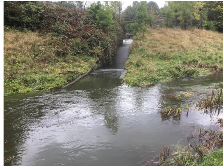
Photo 29: Concrete outfall from Pond D
