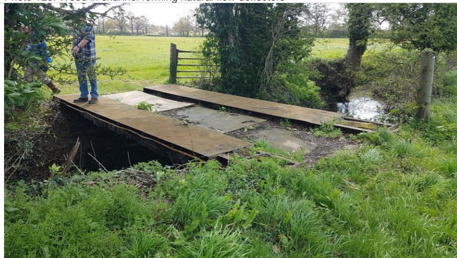
Photo 123: Farm bridge at Brook Farm from left bank
