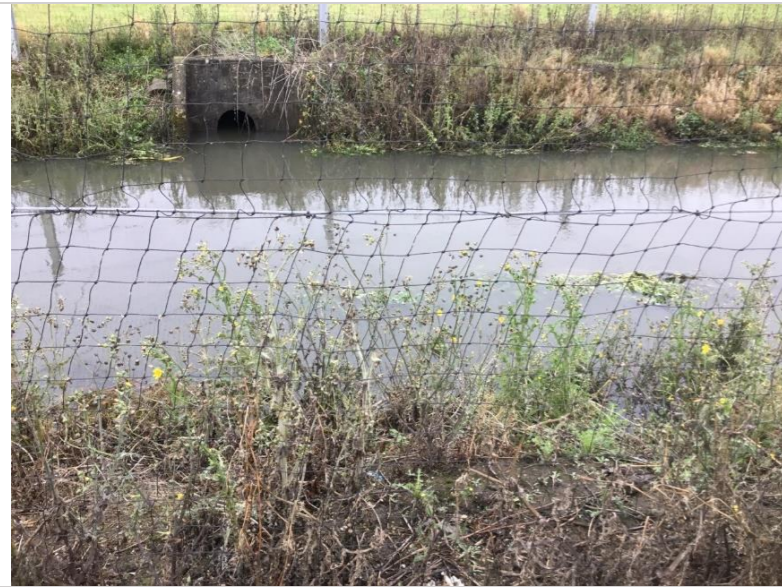
Photo 100: Concrete outfall on left bank
