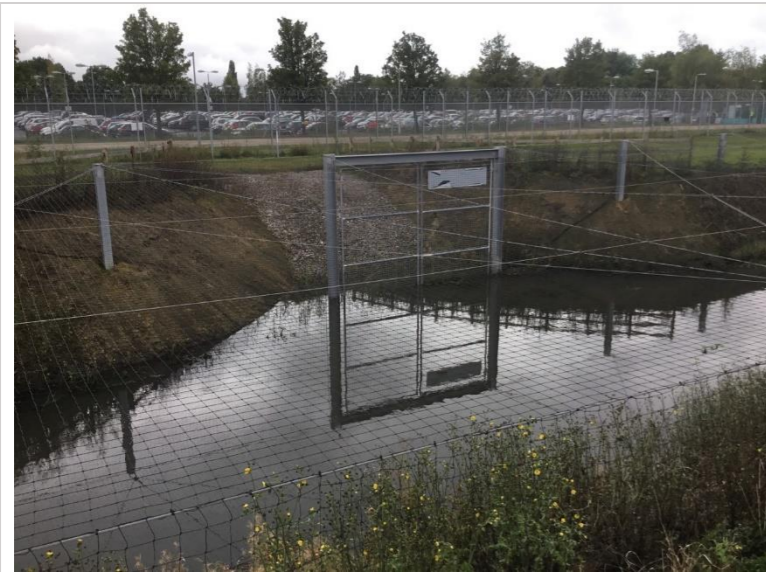
Photo 106: Gravel access path on left bank at Car Park X
