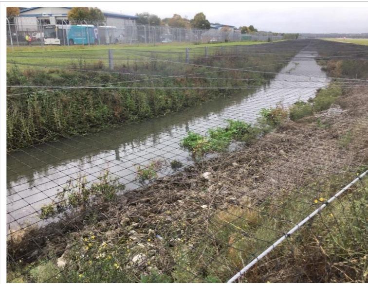
Photo 95: Gabion mattresses on right bank outer meander formed of stone rubble
