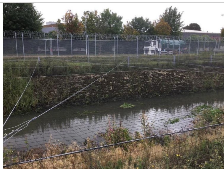
Photo 89: Concrete blockwork bank exposed on left bank
