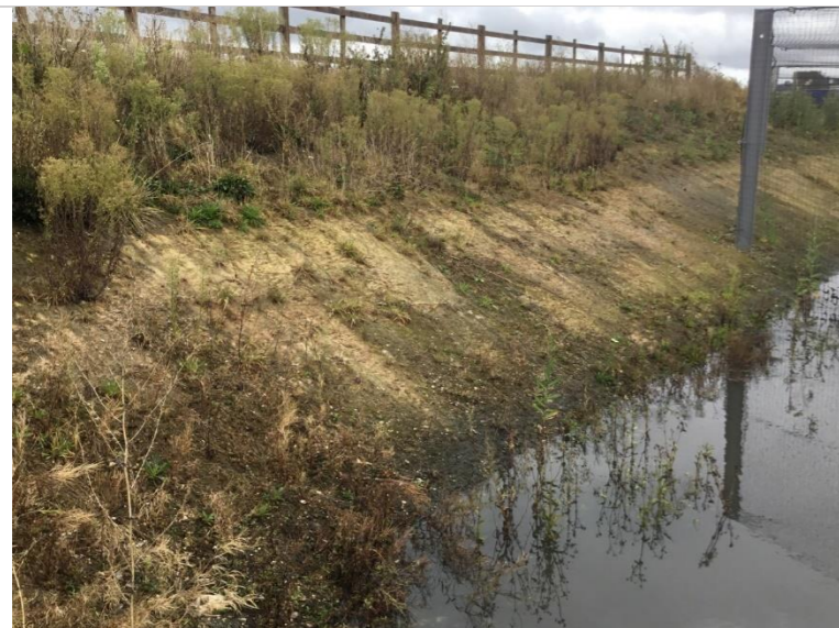
Photo 91: Geotextile over clay banks exposed
